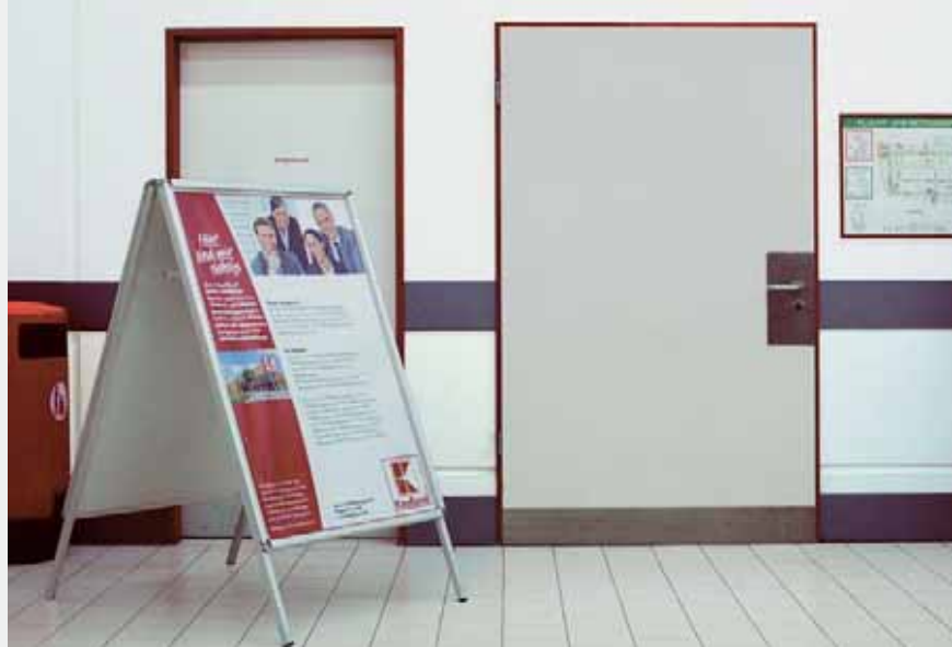
Shopping centre internal door with stainless steel protective plate around the handle and base
